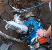
Mill the slot by rotating valve assembly and cutter 120° across the top of the pipe (no coupon, all milling chips removed).
