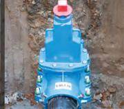
The integral isolation valve allows for removal of the cutter and the installation of the valve bonnet, all under full line pressure.
