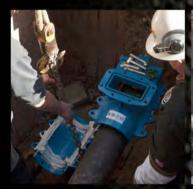
Place and secure the precision machined valve body to the pipe.
