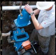
Remove bonnet and install cover plate (under pressure) after use as a line stop.
